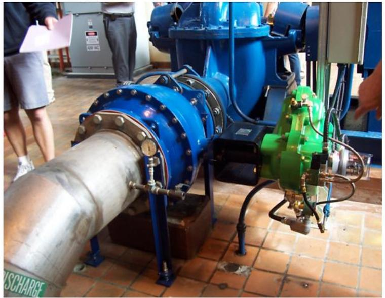
manufacturer for the significant but necessary repairs. Unfortunately, the cost to repair each valve was over half the cost of completely replacing them with new valves. Instead of the costly repairs, the WTP proposed a trial replacement of one of their faulty valves with the Val-Matic® Ener•G® Rubber Seated Ball Valve.
